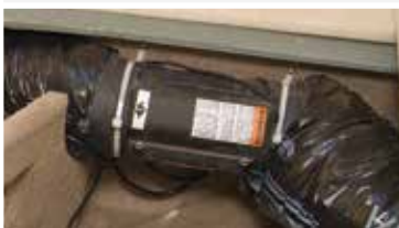
In-duct air purifier installed under a berth within the A/C duct
