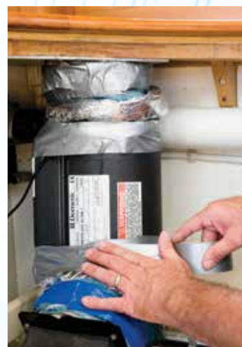
Breathe Easy In-Duct air purifier being installed in an air conditioner duct line
