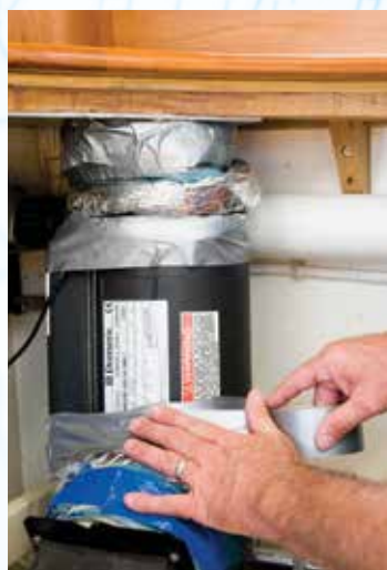
Breathe Easy In-Duct air purifier being installed in an air conditioner duct line
