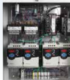
Custom-made fan control enclosure with VFDs
