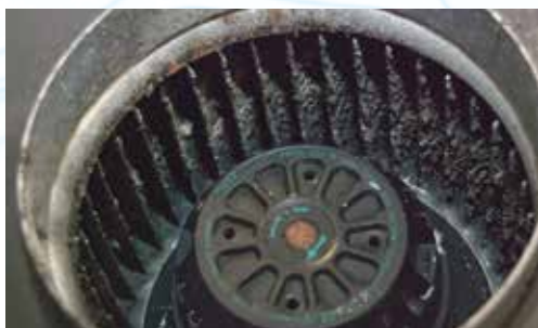
Mold thriving on the A/C blower's fan blades
