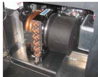
A Cruisair Turbo 16,000 BTU/hr air conditioner installed on a USCG patrol boat by Metal Shark
