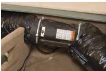
In-duct air purifier installed under a berth within the A/C duct
