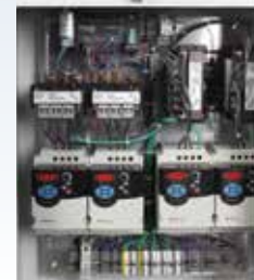
Custom-made fan control enclosure with VFDs
