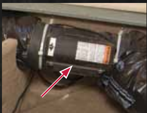
The in-duct Breathe Easy™ Air Purifier installed under a berth within the air conditioner's duct work
